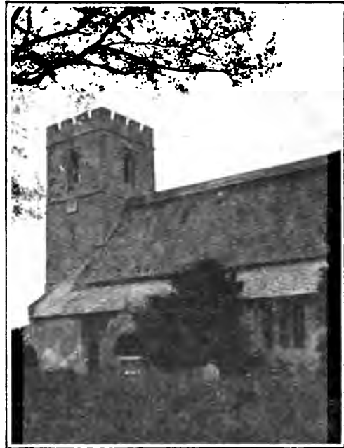
RAMPTON CHURCH, CAMBS., SHOWING THATCHED ROOF OF NAVE (SOUTH ELEVATION).
